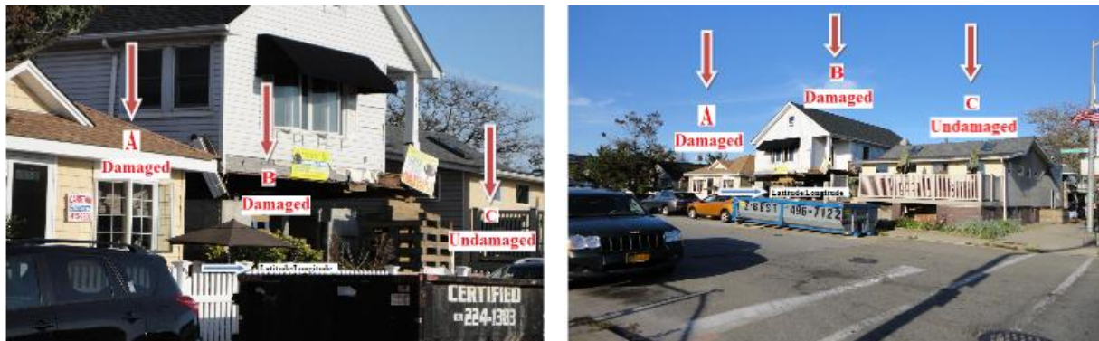
Figure 9. Comparison of damaged and undamaged houses in Long Beach, NY. In the figure, the damaged one, house B, has been raised for repairing.
